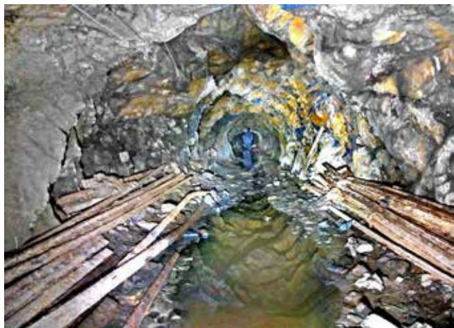
Nigel Ostler-Harris standing at the junction in Robert's level, notice the steel Armtec tunnels to the right which was an open stope to the surface and was previously the only access into the lower workings. The tunnel ahead had previously been filled with rubbish from stope above. Photo Clive Penfold
